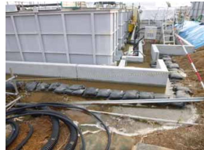
Condition of the overflow (Area (1))
