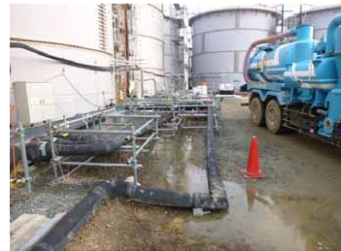
Condition of the overflow (Area (3))
