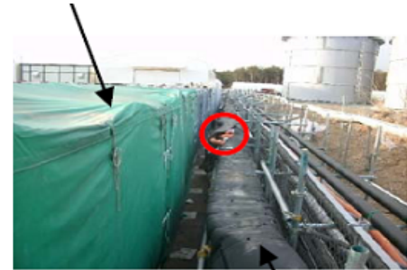
Leakage point on 5 th April
