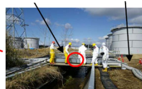
Leakage point on 26 th March
