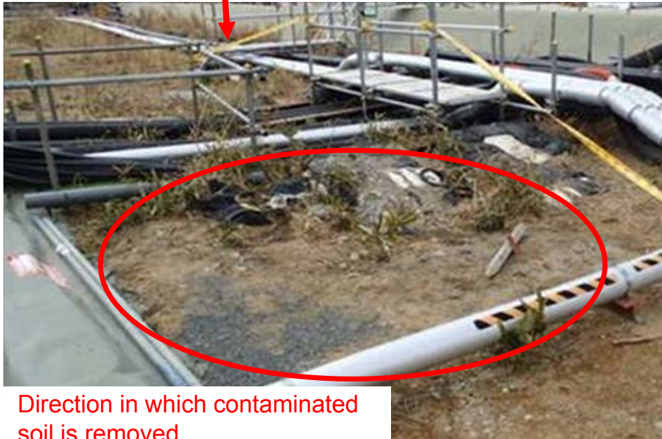
The soil near the surface of the earth is collected manually (combed out) Facing is carried out and cover is installed
