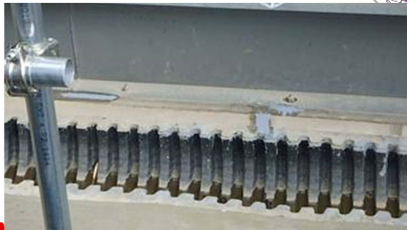
Filling the gaps (3/14 - 3/17)
