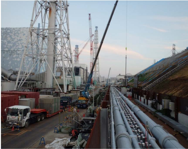
Installation completed on the west side of No. 2-4 buildings
