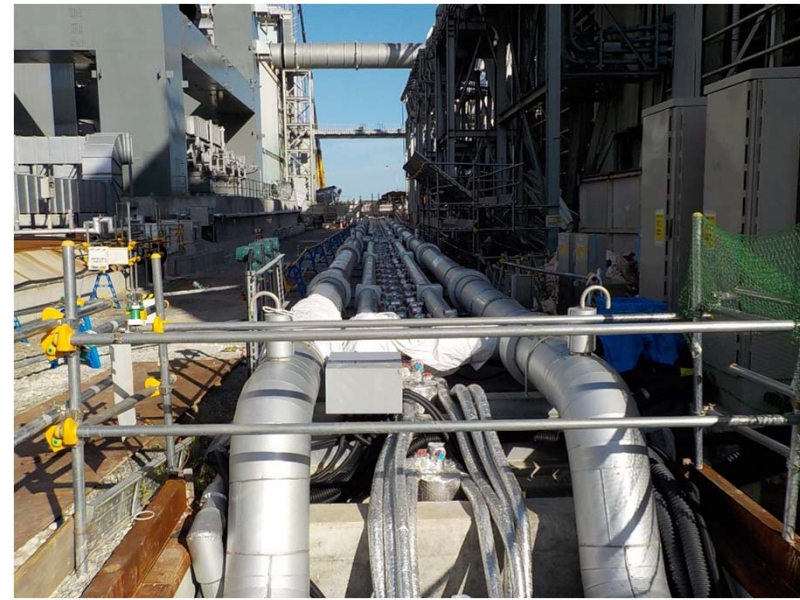
Installation completed on the south side of No. 4 buildings
